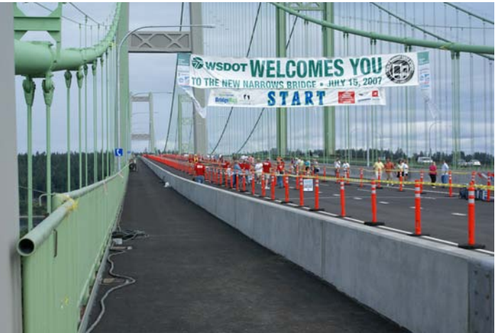
Future Bike/Pedestrian Lane on the New Tacoma Narrows Bridge (Photo submitted by Carla Gramlich)
